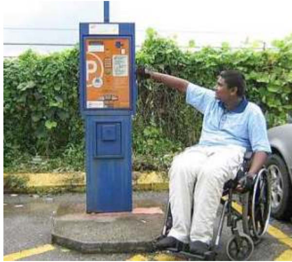
Unreachable: The raised platform at the base of the parking ticket machine makes it impossible to reach from a wheelchair.
