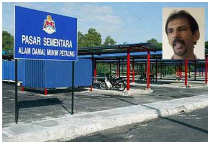
Ready and waiting: The site of the new temporary market in Taman Bukit Anggerik. It is just 200m away from the present market.
